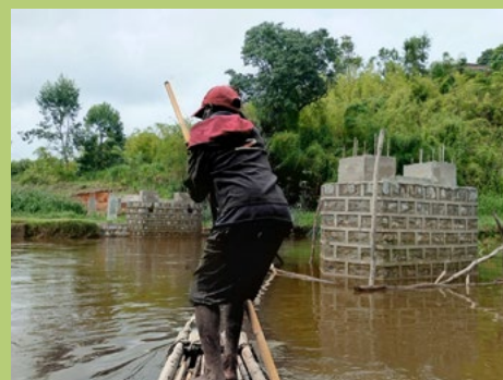
Footbridge being built © IMPACT Madagascar
